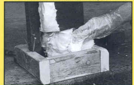
... were completely sawed off and replaced with ...
