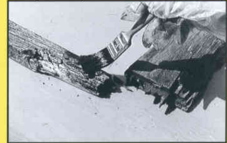
Pouring or brushing is sufficient where absorption is easy
