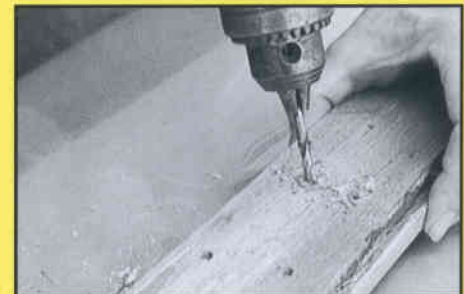
Drilling allows deeper penetration
