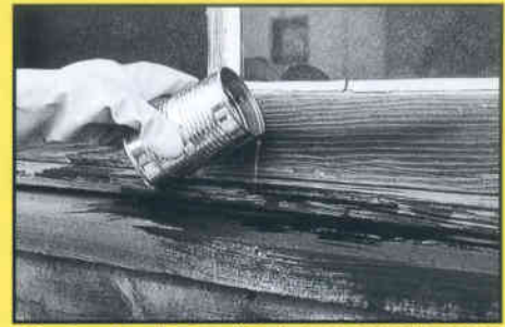
Pouring or brushing is sufficient where absorption is easy
